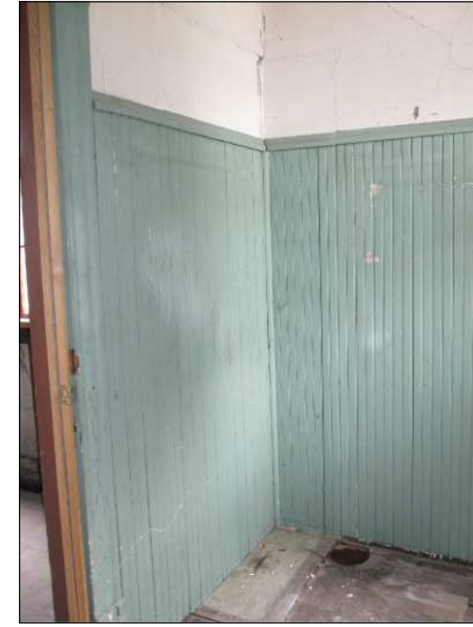
- EXISTING WOOD WAINSCOT PANELS. - NEW WAINSCOT TO MATCH SIMILAR SIZE, STYLE / PROFILE AND DIMENSIONS OF EXISTING PANELS.
