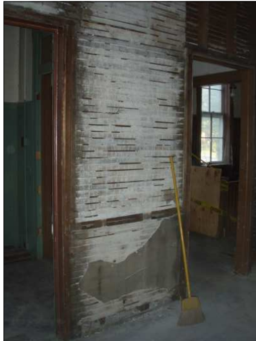
- LOWER HEIGHT OF ORIGINAL WOOD WAINSCOT PANELS IN ORIGINAL CLASSROOM AREA. - PROVIDE GLASS DISPLAY ENCLOSURE, PER OWNER'S REQUIREMENTS. REFER TO KEY NOTE #4R FOR ADDITIONAL INFORMATION.
