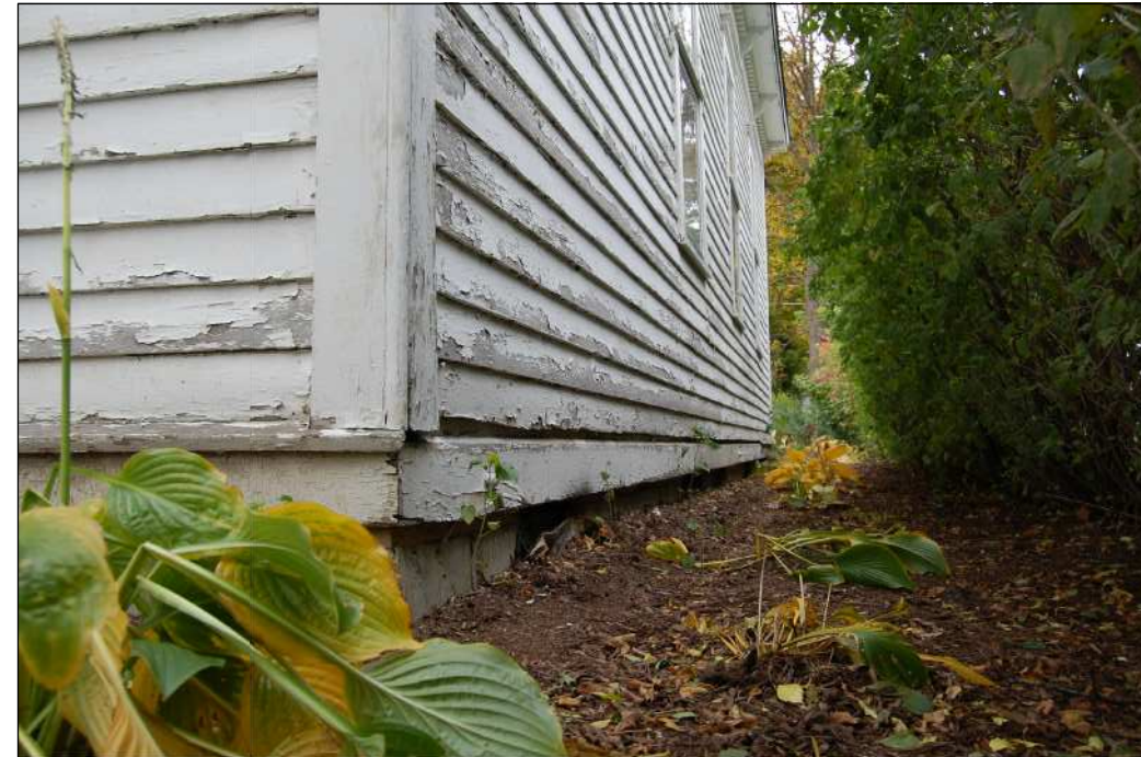
- EXISTING EXTERIOR WOOD BASE TRIM TO BE REPAIRED AND REPLACED AS REQUIRED.
