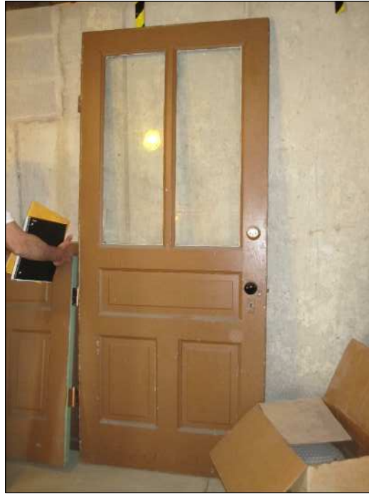
- EXISTING DOOR TO BE REINSTALLED. - NEW DOORS TO MATCH SIMILAR STYLE AND PROFILE OF EXISTING DOOR.
