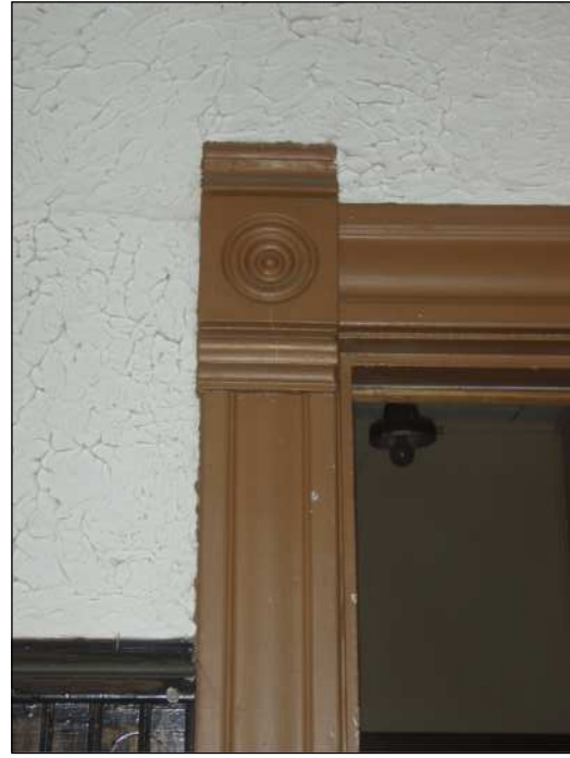
- EXISTING WOOD DOOR ARCHITECTURAL TRIM TO BE REINSTALLED. - NEW TRIM TO MATCH SIMILAR STYLE AND PROFILE OF EXISTING TRIM.
