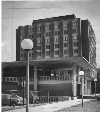
Stanley R. Pierce Tower shortly after its dedication in 1963.
