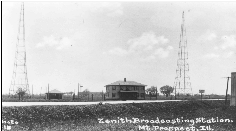
The station and towers at Rand and Central Roads.
